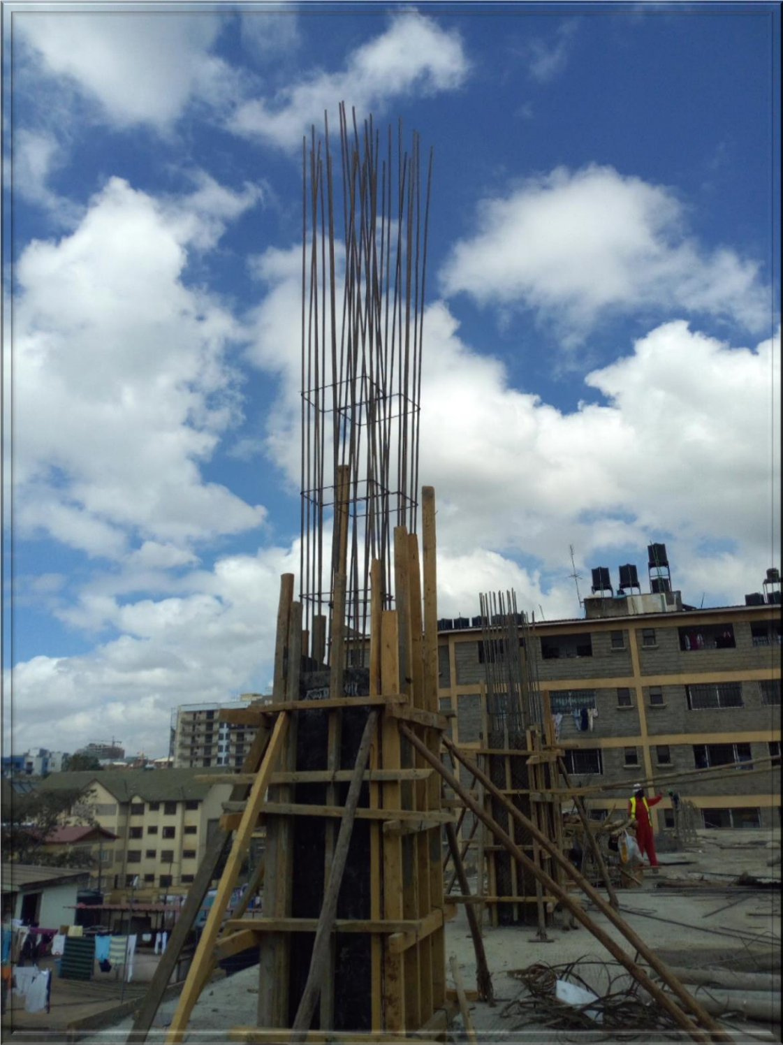
Fig. 06. Concreting works progressing on as below
