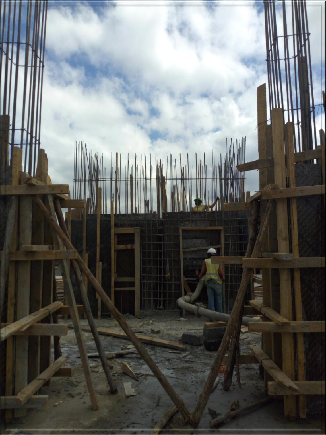
Fig. 04. Lift shaft construction in progress
