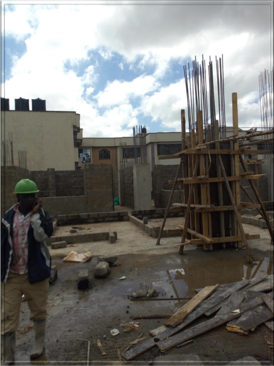
Fig. 05. Concreting and columns works progressing on as below
