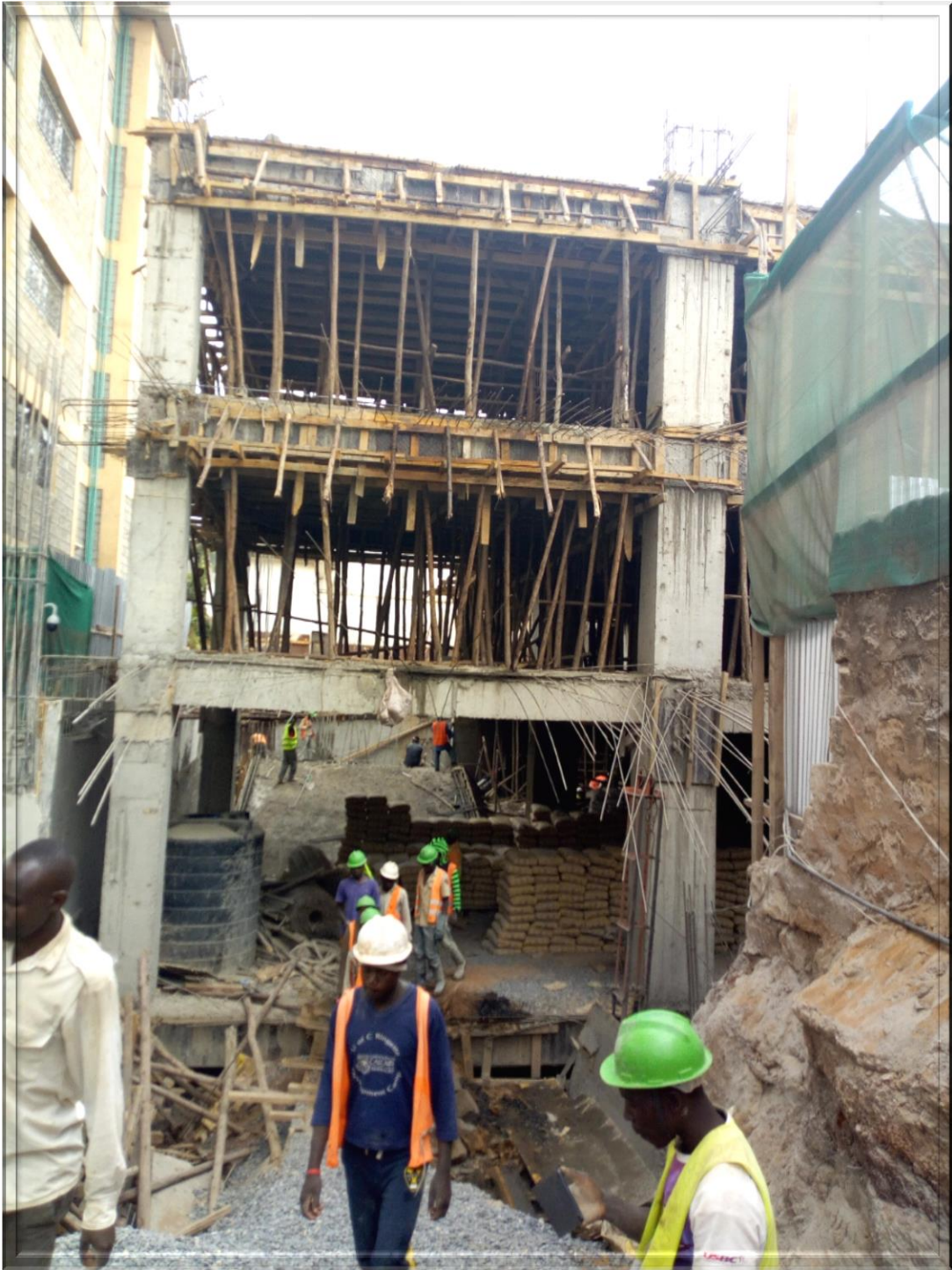
Fig. 01. Construction works progress as per the picture below
