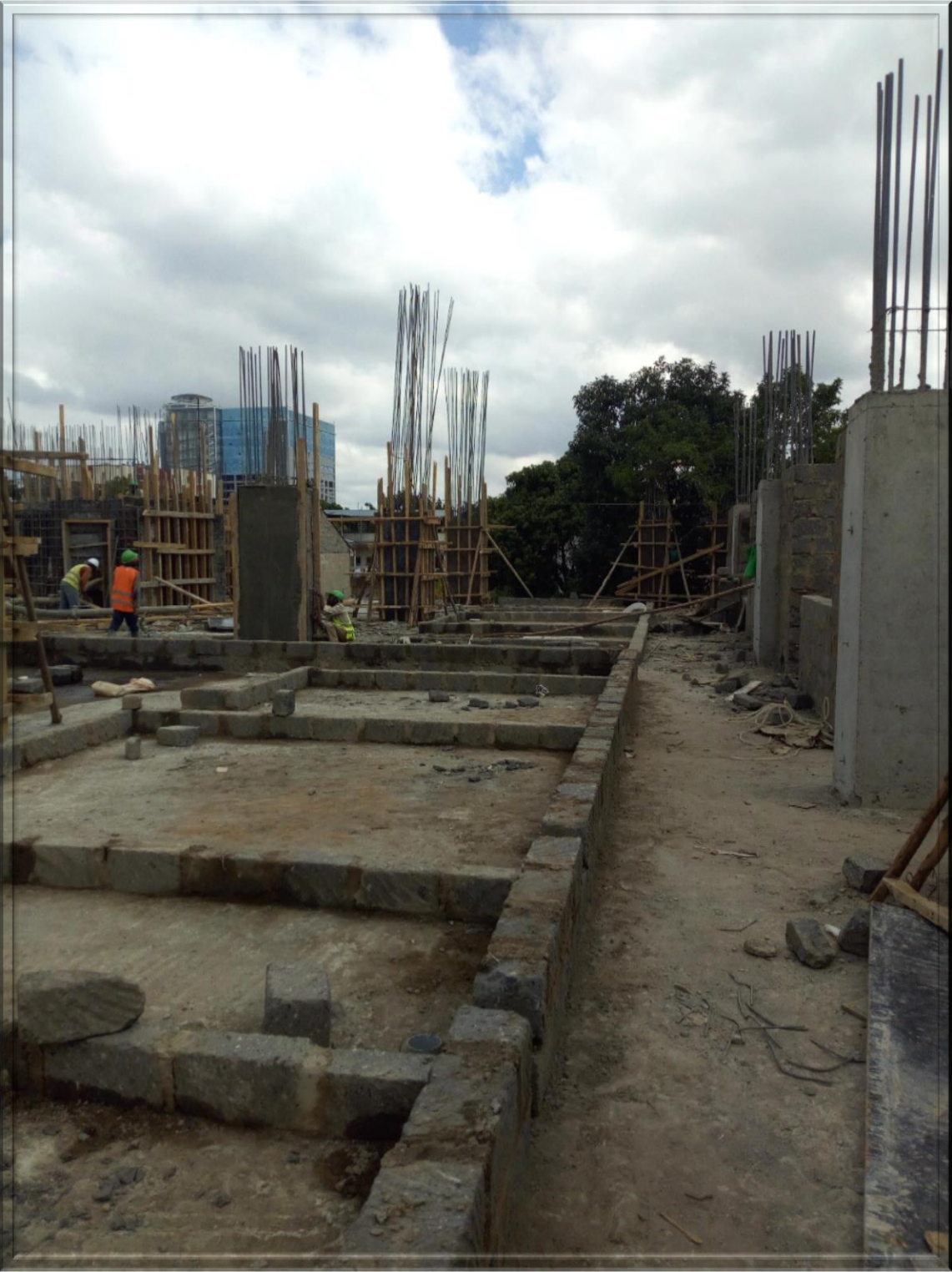
Fig. 03. Excavations works going on as below
